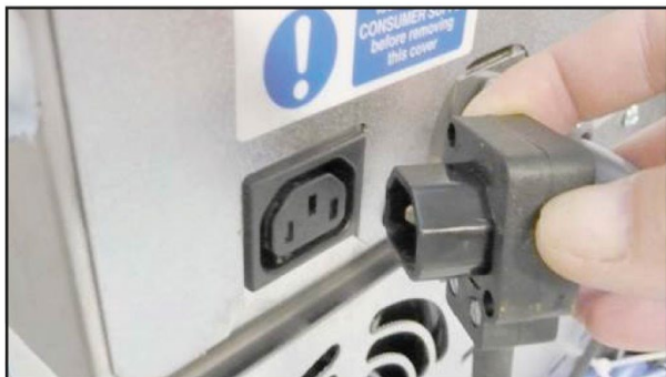
Figure 46: Plugging in the condenser unit
