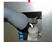
OVEN DRAINAGE CONNECTION AT REAR
