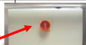
PROVER MAIN ISOLATOR
