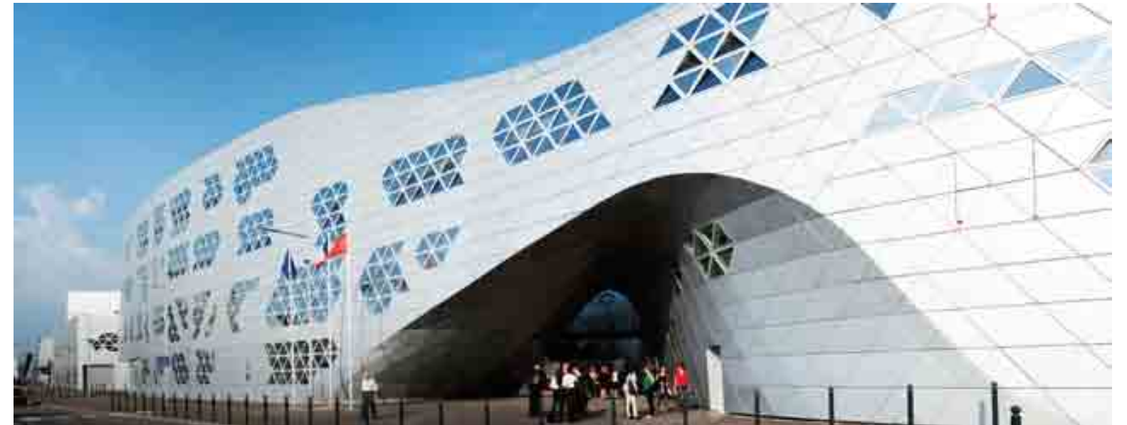
The futuristic project for the Lycée Georges Frêche was designed by Massimiliano Fuksas.
