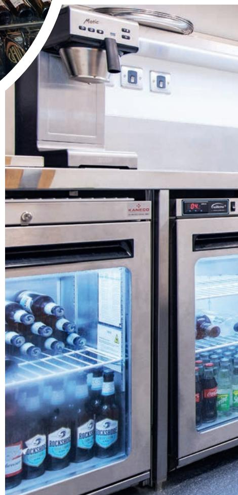
factor with practical features – it's a pass-through unit displaying chilled wines, it has a double aspect so it can supply both bars, and it also runs off the chilled-water system.
