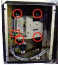
Unplug the HMI power cable and remove the old HMI by loosening and removing the 4x retaining clips with a small posidrive/flat head screwdriver. Then push the HMI out of the cut out.
