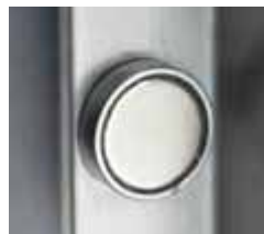
Magnets allow the external window to open easily
