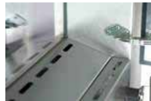
Thanks to its slanting sills, the space between the two windows helps reduce the accumulation of residue and allows perfect cleaning.
