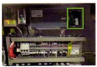
Fix the M251 to the DIN rail – ensure that the 3x retaining clips are in the out position before offering up to the DIN rail, then use a screwdriver to push the 3x retaining clips in – ensure it is mounted securely.
