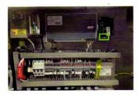
Connect the power supply plug to the M251 (connector at bottom). Note the retaining shroud hinges up to enable the connector to be inserted, insert then hinge the shroud down to fully engage.
