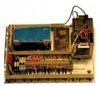
Remove the I/O connector from the TLCC (pull to remove). Trace the wires back to the terminals (I02 to I08) and remove using a small screwdriver. Trace the wire back to the emergency stop relay (I01) and remove with a small screwdriver.
