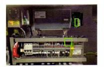
Connect the CAN cable to the port at the top of the M251. Connect the wires at the other end of this cable to the terminals with the corresponding wire numbers (to the same location as the ones previously removed)
