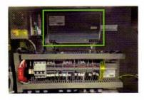
Fix the 36 Volt power supply onto the DIN rail – ensure it is mounted securely.
