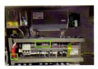
Connect the wires at the other end of the IO cable to the terminals with the corresponding wire numbers (to the same location as the ones previously removed) for wires IO1 to IO7 and OV. Connect IO0 to the emergency stop relay connection point 14.
