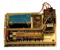
Remove wires to the power supply of the TLCC using a small screwdriver.
