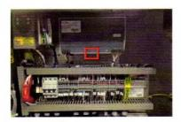
Release the 36 Volt power supply from the DIN rail by using a large flat head screwdriver to pull down on the retaining clip. Lift the power supply off the DIN rail.
