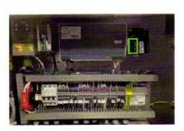
Connect the HMI cable to one of the connectors marked ETHERNET. Ensure that the cable is pushed in firmly, you should hear a "click".
