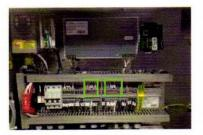
Connect the wires at the other end of the power cable to the terminals with the corresponding wire numbers (to the same location as the ones previously removed).
