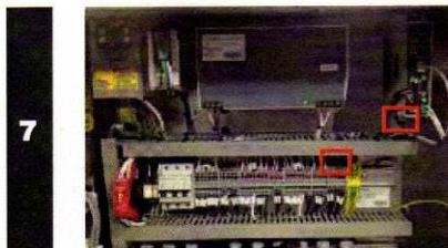
Remove the 'D' connector from the bottom of the LMC20 by pulling the connector. Trace the wires back to the terminals (C+ / C-) and remove using a small screwdriver.
