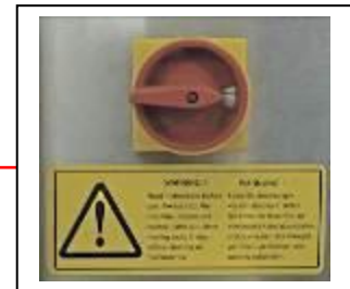
MAINS SUPPLY ISOLATOR
