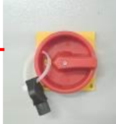
MAINS SUPPLY ISOLATOR
