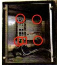
Fit the new HMI (HMIGTO3210) using the 4x retaining clips supplied in the box with a small posidrive/flat head screwdriver. Then plug in the power connector.
