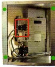
Remove the 'D' connector from the HMI using a small screwdriver.
