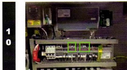
10 Connect the wires at the other end of the power cable to the terminals with the corresponding wire numbers (to the same location as the ones previously removed).
