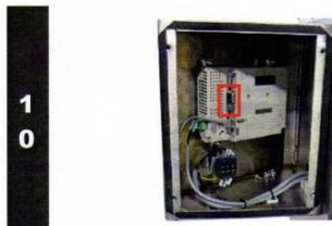
10 Remove the Modbus cable from the COM1 connector on the HMI by using a small screw driver to loosen the fastening screws and then pulling to release.
