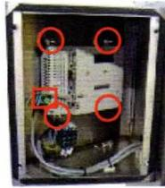
Unplug the HMI power cable and remove the old HMI by loosening and removing the 4x retaining clips with a small posidrive/flat head screwdriver. Then push the HMI out of the cut out.
