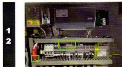
12 Connect the wires at the other end of the IO cable to the terminals with the corresponding wire numbers (to the same location as the ones previously removed) for wires I01 to I07 and 0V. Connect I00 to the emergency stop relay connection point 14.
