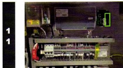
11 Connect the IO cable plug to the M251 expansion module at the right. Push the connector into the housing – ensure it is fully engaged.
