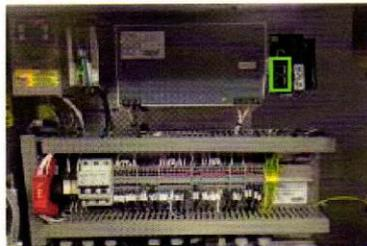
Connect the HMI cable to one of the connectors marked ETHERNET. Ensure that the cable is pushed in firmly, you should hear a "click".
